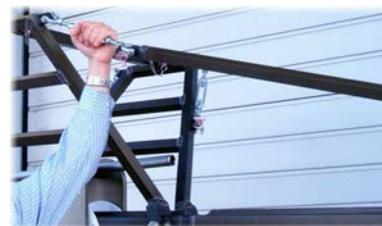
Tensioning the turnbuckle
